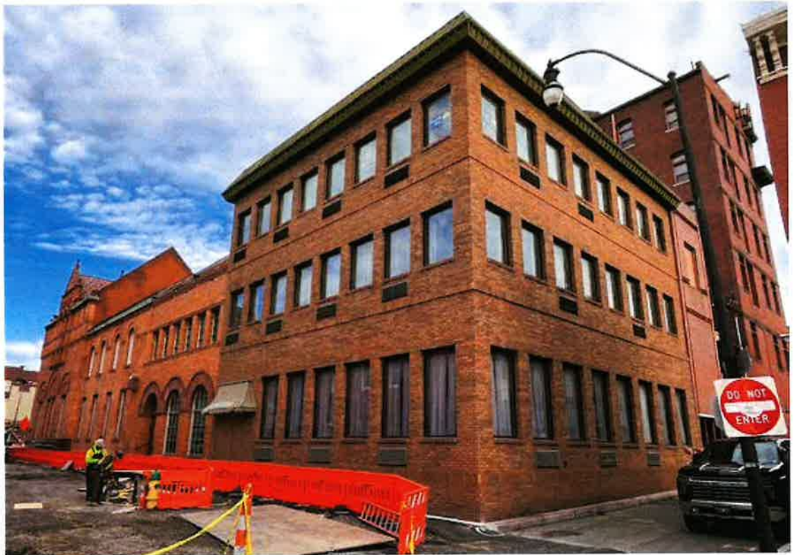
E-13 Liberty Street and Pershing Street Corner_2023_12
