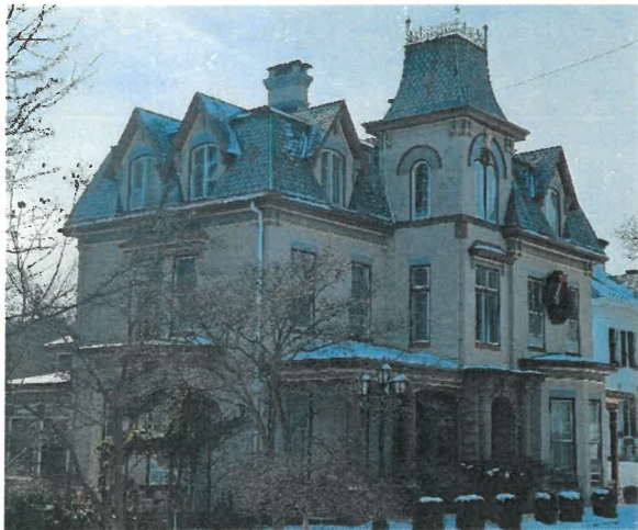
Photos 40 & 41: 522 Washington St – Owens Corning Duration
