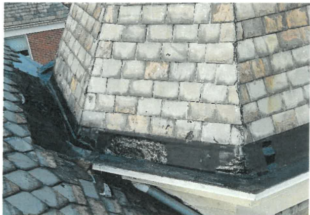
Photo 20: Turret gutter liner
