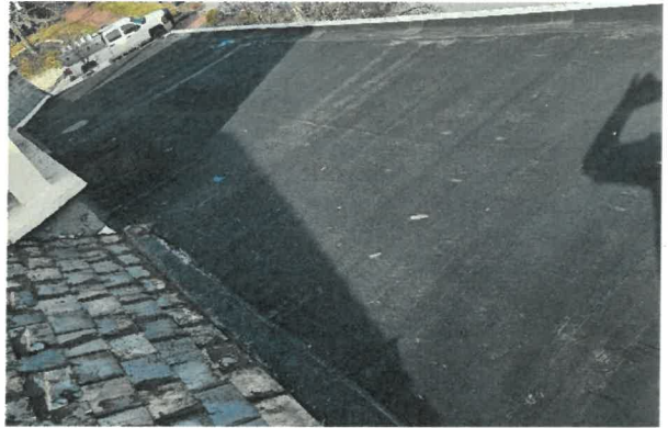
Photo 18: Flat roofing front
