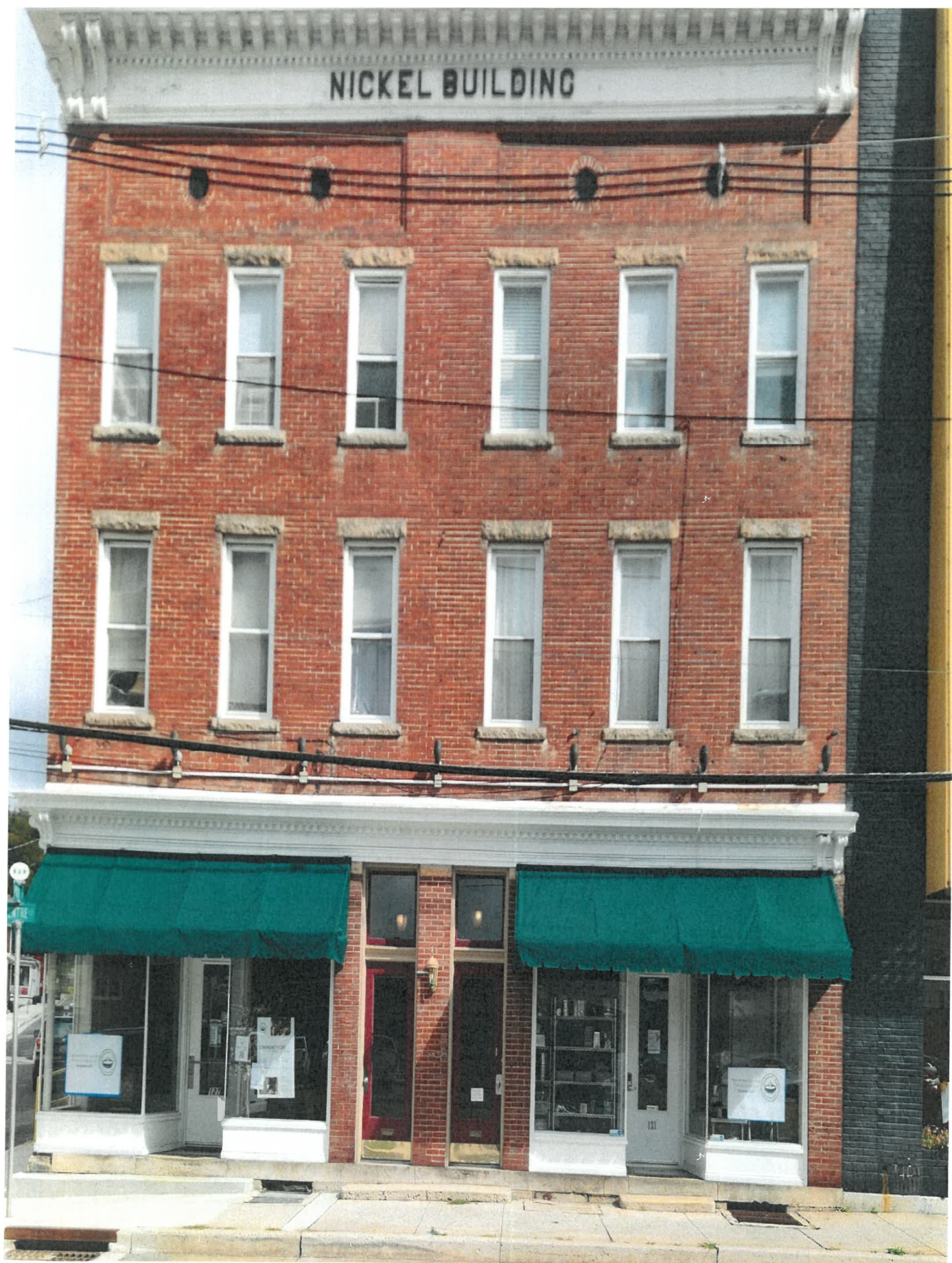
Bldg with Lumark TCRL15M lights
