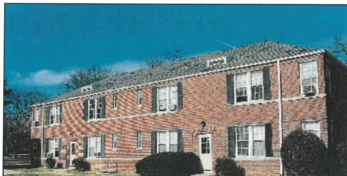
Typical view of Colonial-Revival apartment building in complex before rehabilitation. Note the mottled appearance of original slate due to numerous past repairs.
