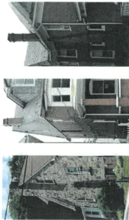
Guideline 21: Does your building or building type have a chimney where the entire chimney form is on the exterior end of the building (left)? Is it on the interior end of the building, where nothing but the top is visible (middle)? Or somewhere in between (right)? Is it in the middle of the building? These characteristics are part of the overall design of the building and should be maintained.
