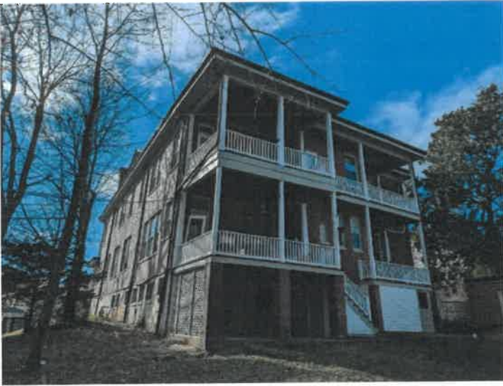
Exterior Evaluation / Exterior Home Structure Walls
