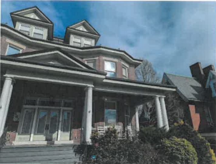
Exterior Evaluation / Exterior Home Structure Walls
