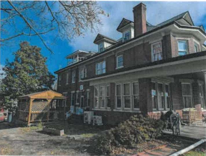
Exterior Evaluation / Exterior Home Structure Walls
