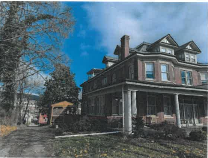
Exterior Evaluation / Exterior Home Structure Walls
