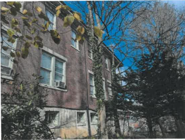
Exterior Evaluation / Exterior Home Structure Walls
