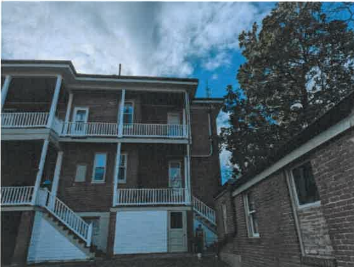
Exterior Evaluation / Exterior Home Structure Walls
