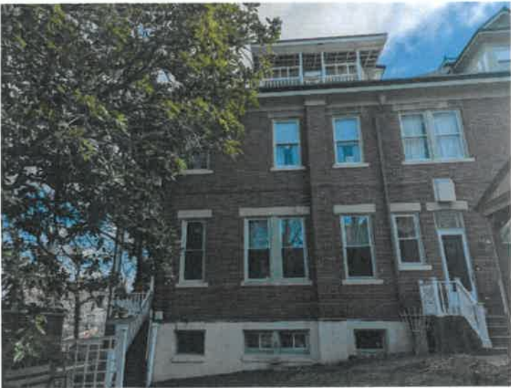
Exterior Evaluation / Exterior Home Structure Walls
