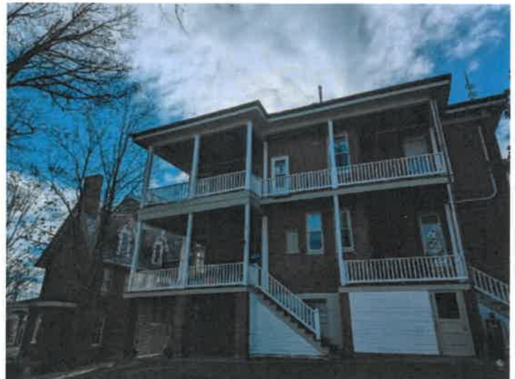
Exterior Evaluation / Exterior Home Structure Walls
