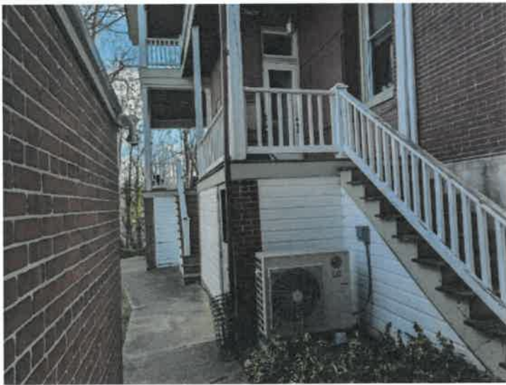
Exterior Evaluation / Exterior Home Structure Walls
