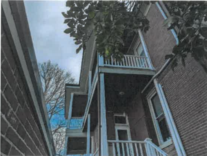
Exterior Evaluation / Exterior Home Structure Walls
