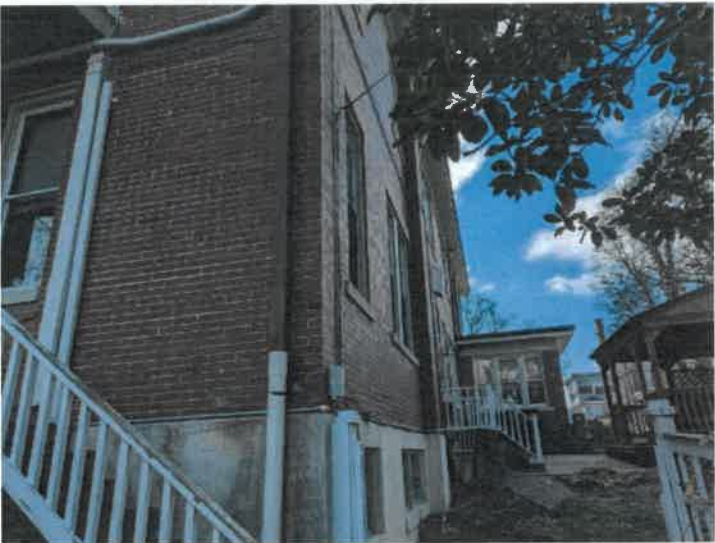
Exterior Evaluation / Exterior Home Structure Walls
