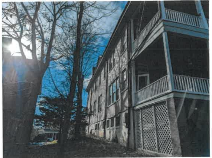
Exterior Evaluation / Exterior Home Structure Walls
