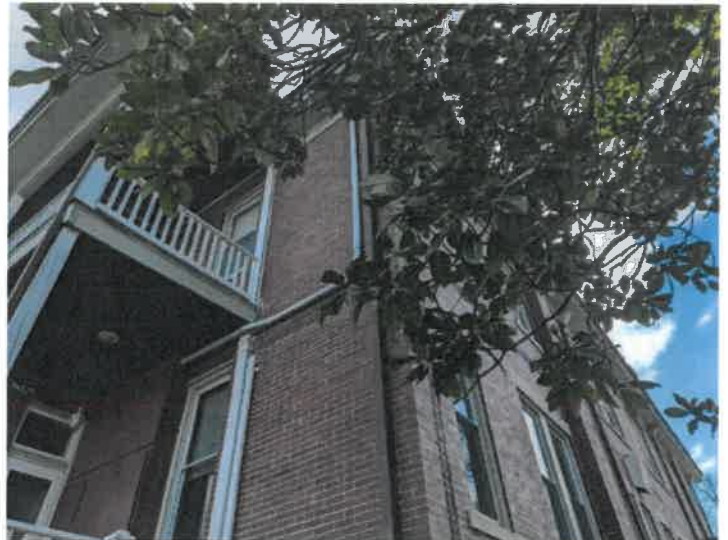
Exterior Evaluation / Exterior Home Structure Walls
