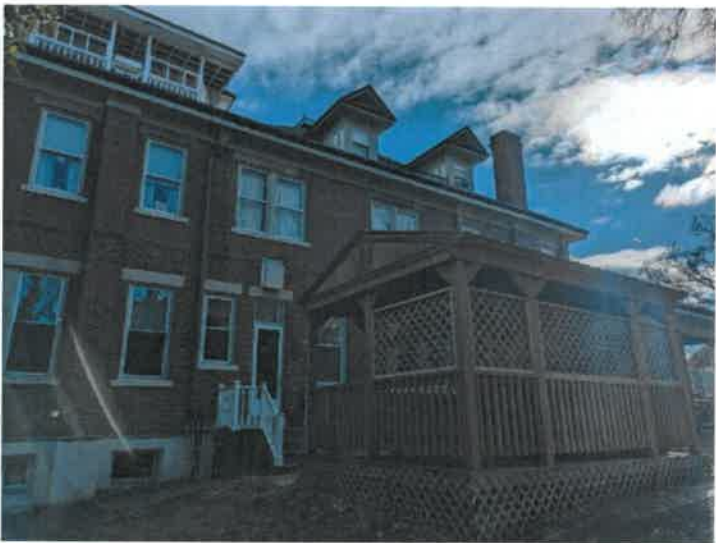
Exterior Evaluation / Exterior Home Structure Walls
