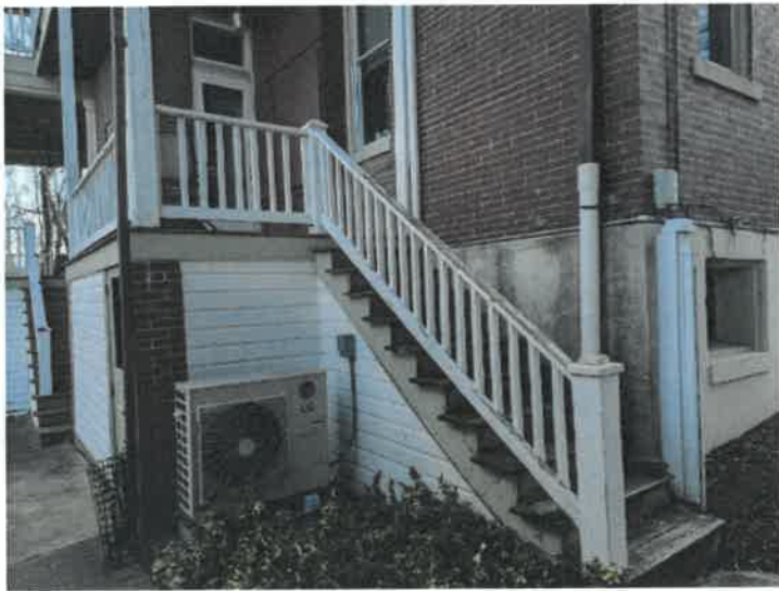
Exterior Evaluation / Exterior Home Structure Walls
