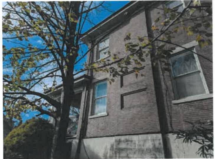
Exterior Evaluation / Exterior Home Structure Walls
