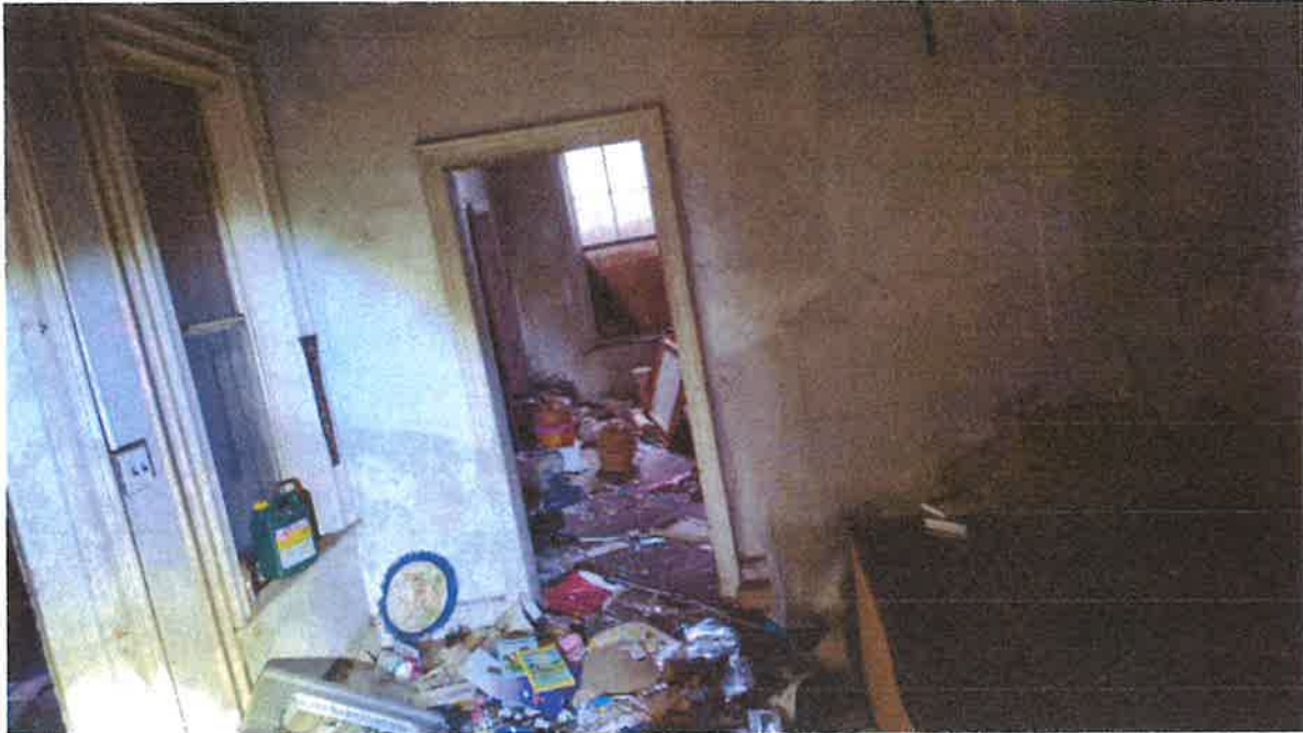
Photo 6. This is looking east on the first floor. The floor was unstable and not safe to walk on.
