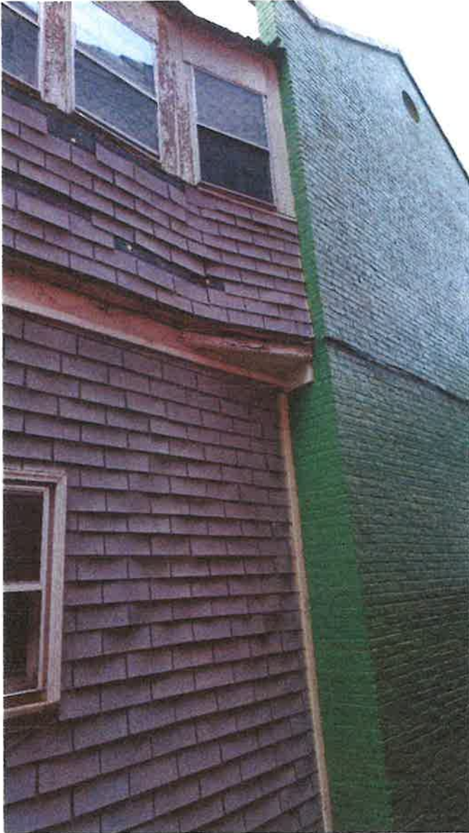
Photo 3. This is part of the north side of 111 Hanover. The shingled walls are the enclosed porch.
