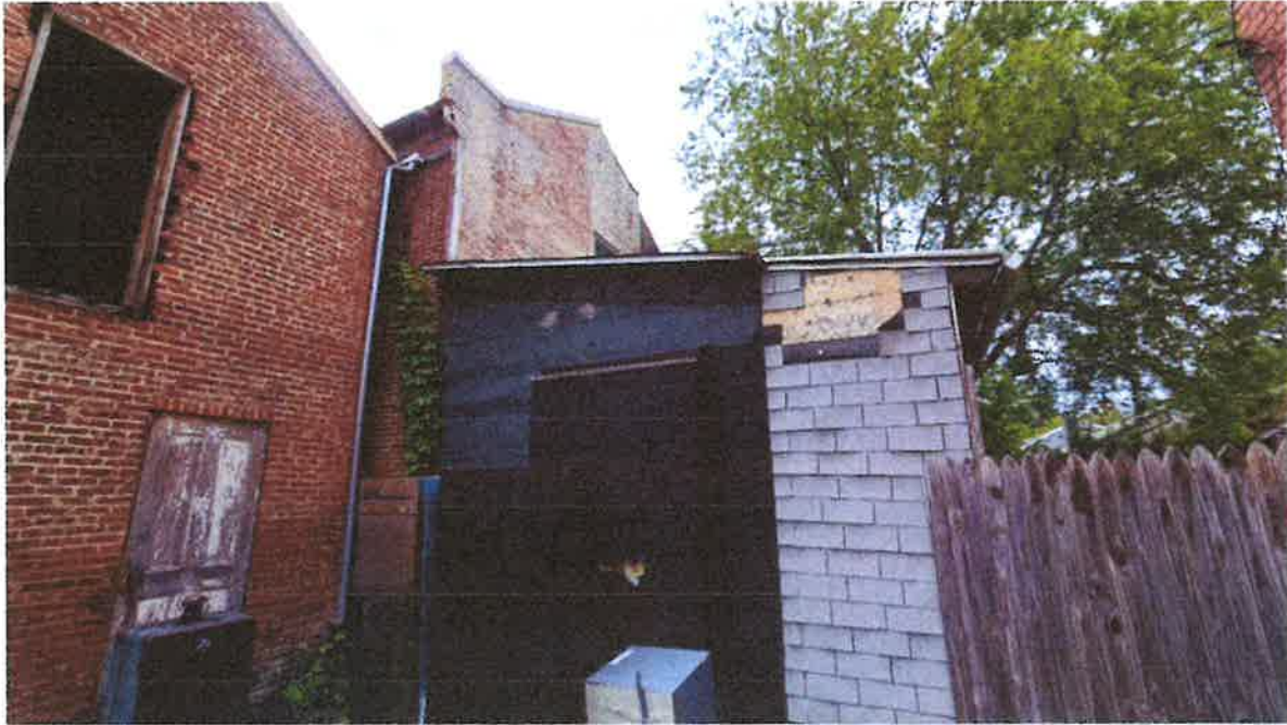
Photo 2. This is the rear portion of 107-109 and 111 Hanover. The shed roof addition is part of 111 Hanover.
