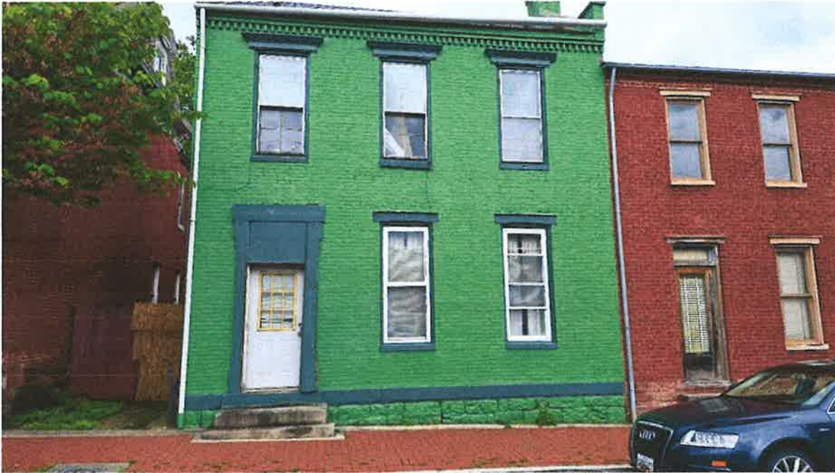
Photo 1. This is the front (west) side of 111 Hanover Street.
