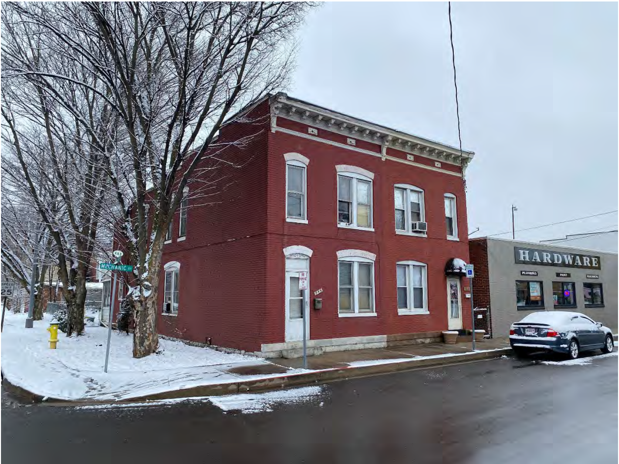
MD-Allegany_Cumberland Downtown Historic District Boundary Expansion_022 Photo 22 of 75. View of 243-245 North Mechanic Street, looking east-southeast.
