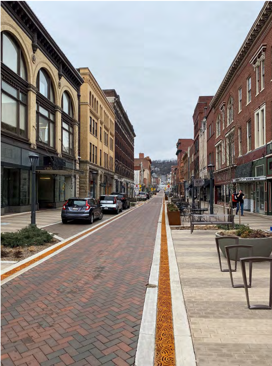
MD-Allegany_Cumberland Downtown Historic District Boundary Expansion_031 Photo 31 of 75. View to the east along Baltimore Street.
