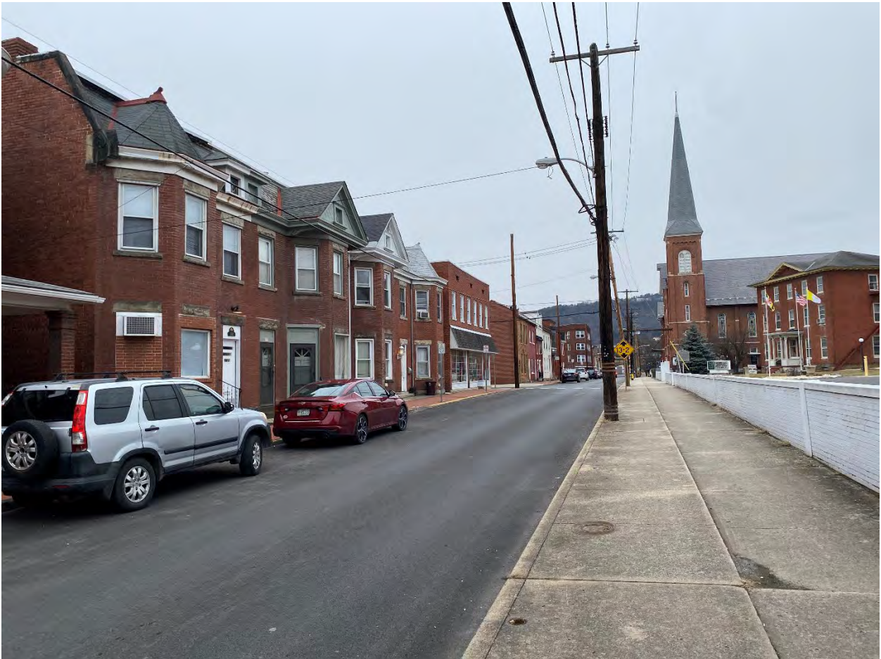
MD-Allegany_Cumberland Downtown Historic District Boundary Expansion_074 Photo 74 of 75. View to the south along North Centre Street.
