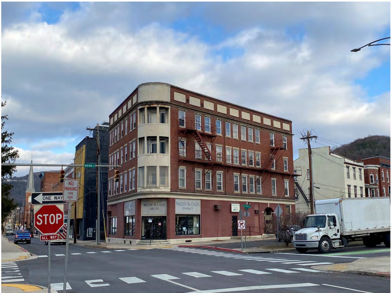
MD-Allegany_Cumberland Downtown Historic District Boundary Expansion_040 Photo 40 of 75. View of 101 Bedford Street, looking north-northwest.
