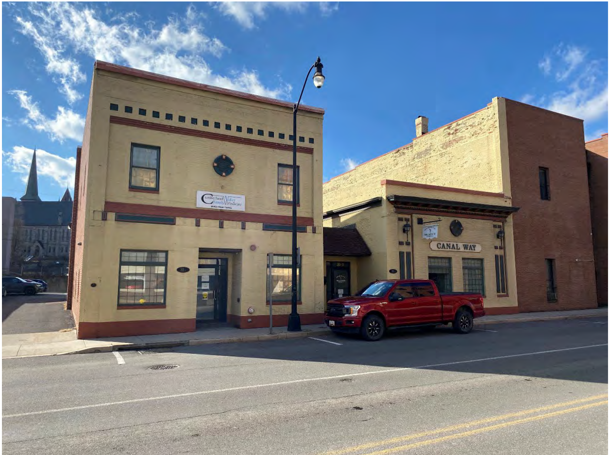
MD-Allegany_Cumberland Downtown Historic District Boundary Expansion_028 Photo 28 of 75. View of 30 North Mechanic Street, looking west-northwest.
