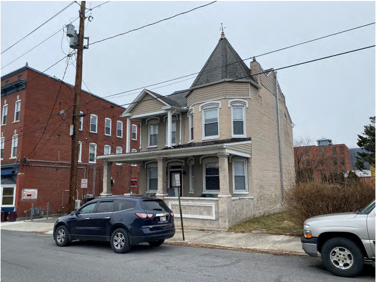
MD-Allegany_Cumberland Downtown Historic District Boundary Expansion_007 Photo 7 of 75. View of 132 Bedford Street, looking southwest.
