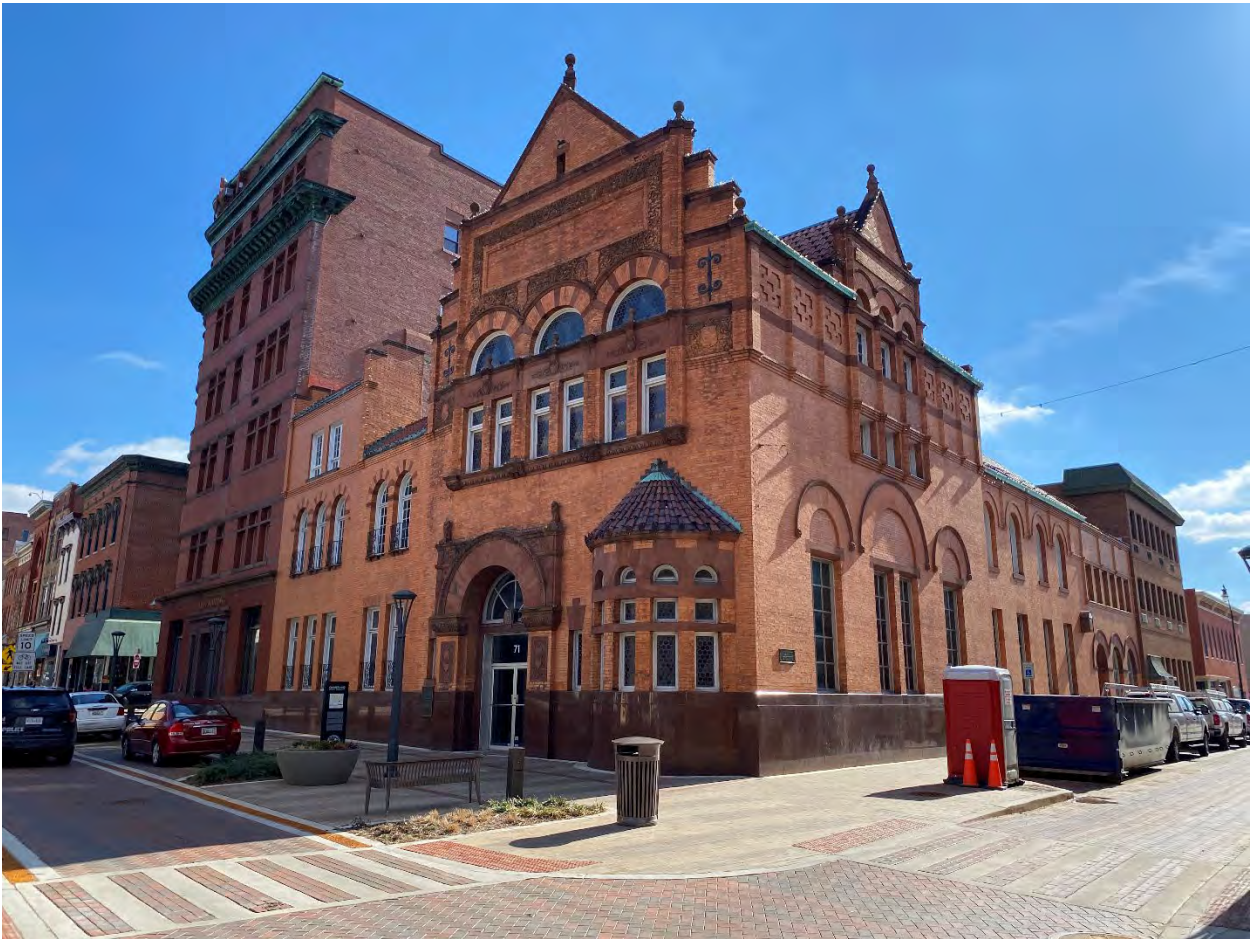
MD-Allegany_Cumberland Downtown Historic District Boundary Expansion_012 Photo 12 of 75. View of 71-73 Baltimore Street, looking southeast.
