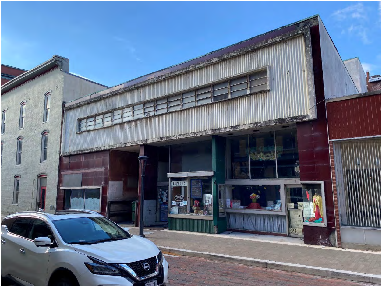
MD-Allegany_Cumberland Downtown Historic District Boundary Expansion_050 Photo 50 of 75. View of 14 North Centre Street, looking south-southwest.
