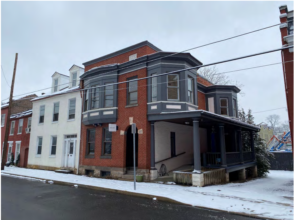
MD-Allegany_Cumberland Downtown Historic District Boundary Expansion_044 Photo 44 of 75. View of 208 North Centre Street, looking south-southwest.
