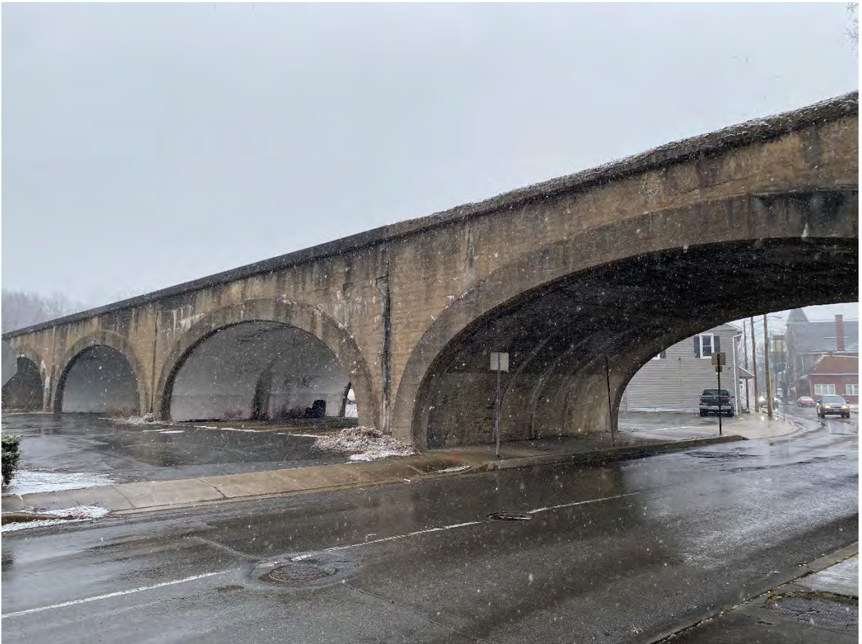
MD-Allegany_Cumberland Downtown Historic District Boundary Expansion_014 Photo 14 of 75. View of B&O Viaduct, looking west.
