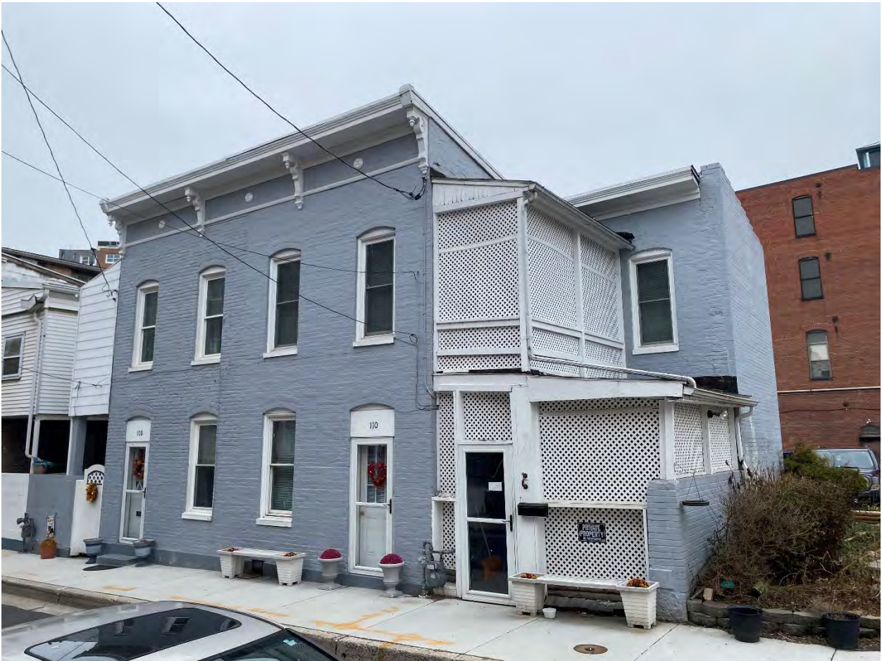
MD-Allegany_Cumberland Downtown Historic District Boundary Expansion_033 Photo 33 of 75. View of 108-110 Polk Street, looking west-southwest.
