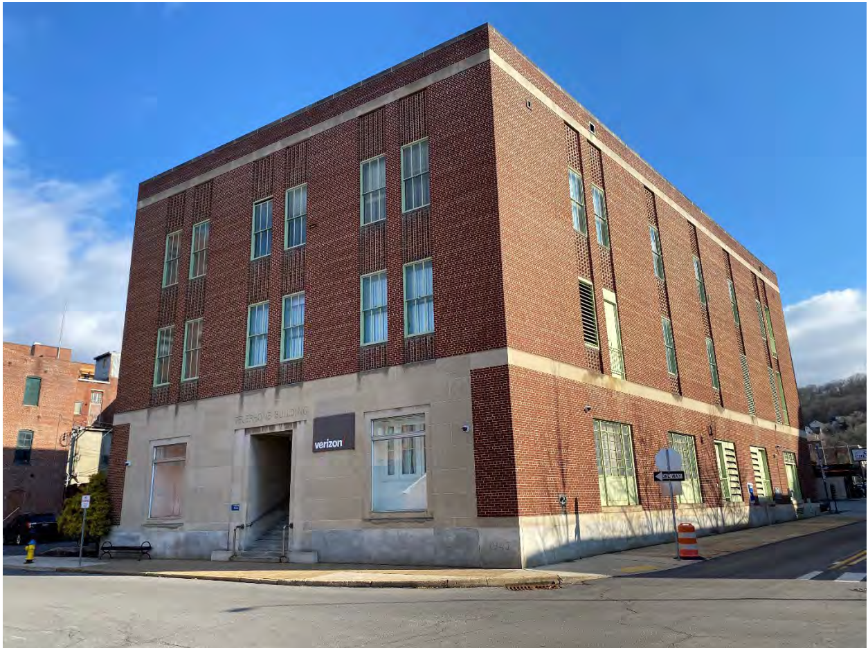
MD-Allegany_Cumberland Downtown Historic District Boundary Expansion_056 Photo 56 of 75. View of 24 South Centre Street, looking northeast.
