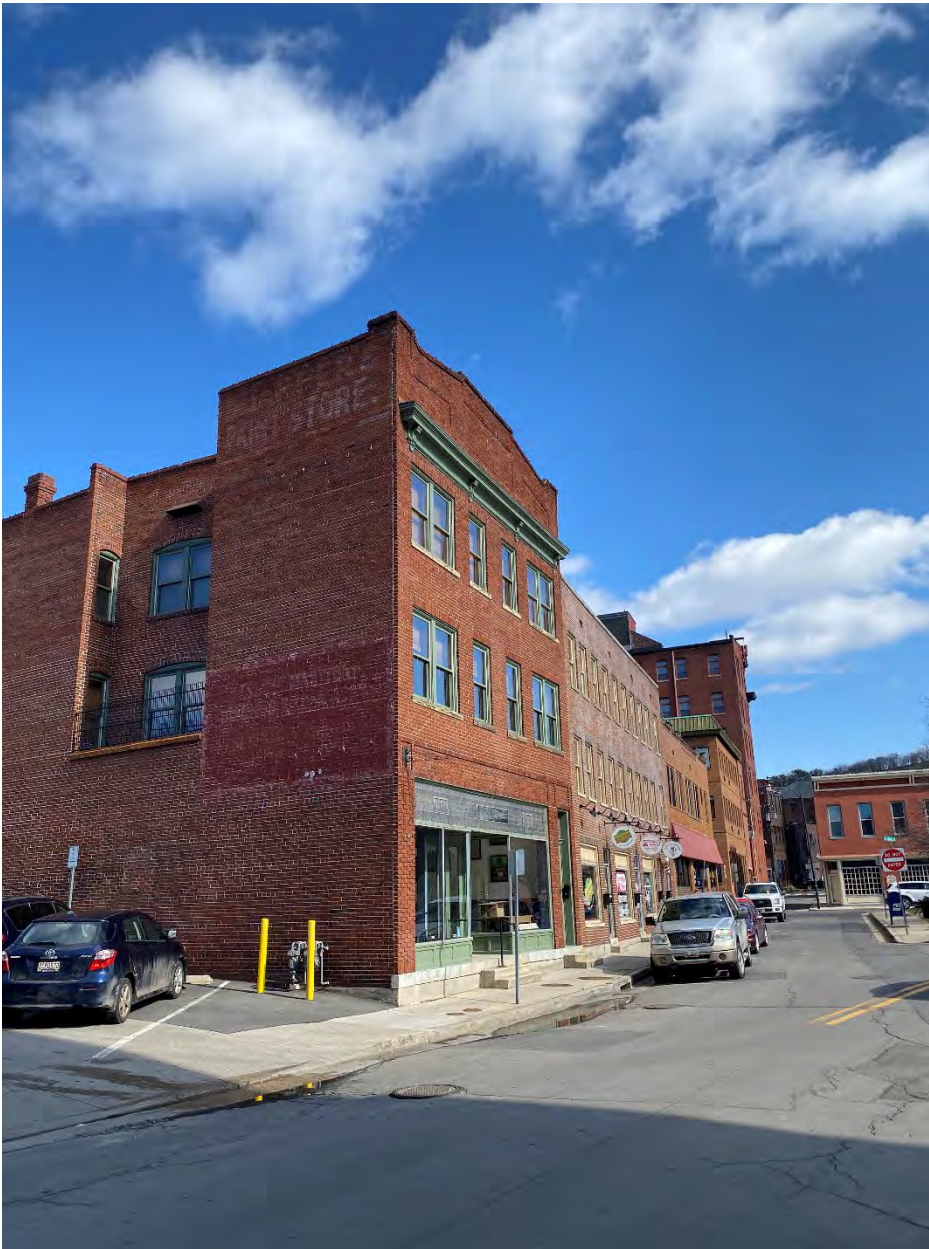
MD-Allegany_Cumberland Downtown Historic District Boundary Expansion_068 Photo 68 of 75. View to the east along Pershing Street.
