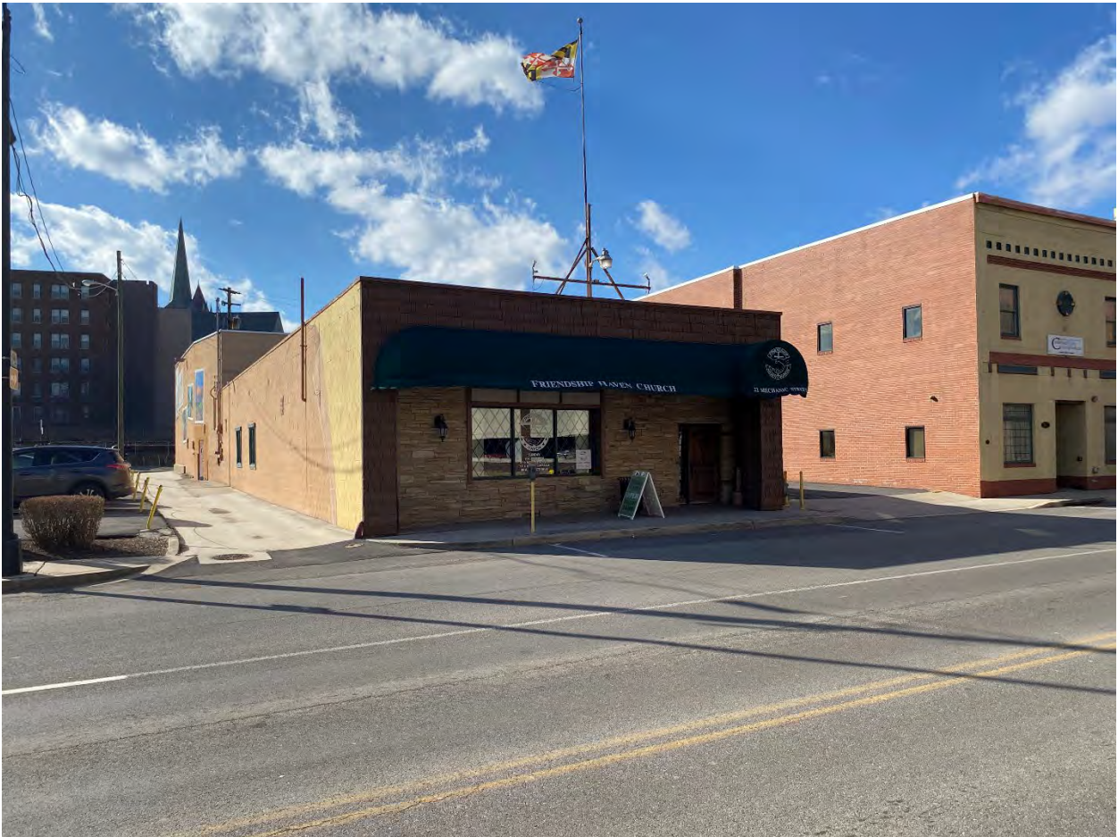
MD-Allegany_Cumberland Downtown Historic District Boundary Expansion_073 Photo 73 of 75. View of 22 North Mechanic Street, looking west-northwest.
