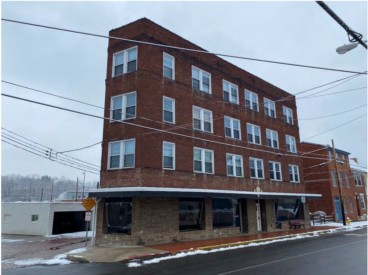
MD-Allegany_Cumberland Downtown Historic District Boundary Expansion_039 Photo 39 of 75. View of 228 North Centre Street, looking west.
