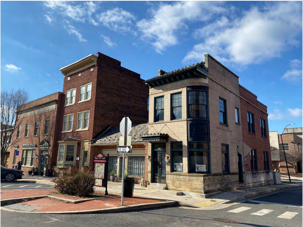
MD-Allegany_Cumberland Downtown Historic District Boundary Expansion_057 Photo 57 of 75. View of 101-107 South Centre Street, looking southwest.
