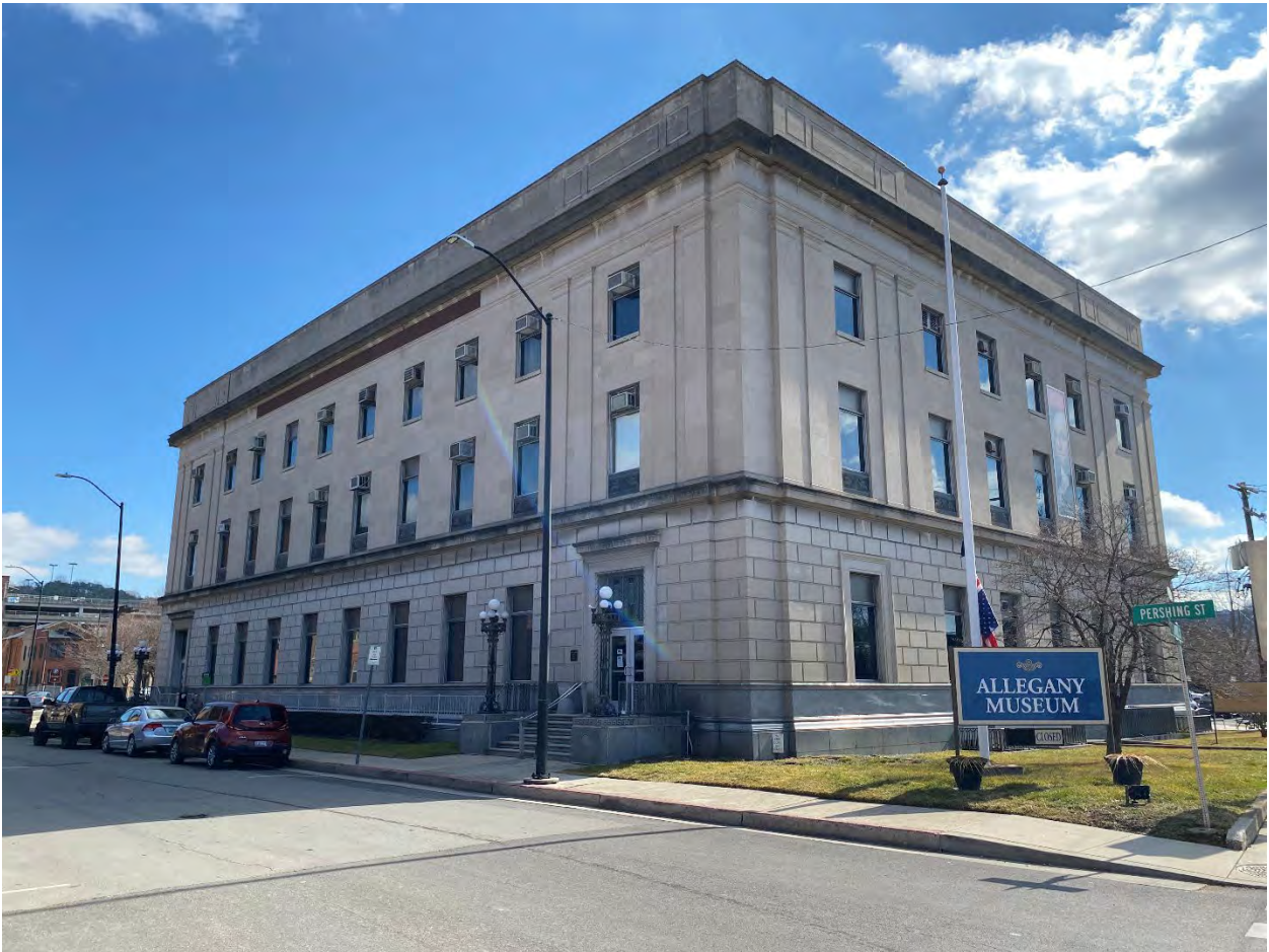
MD-Allegany_Cumberland Downtown Historic District Boundary Expansion_009 Photo 9 of 75. View of 3 Pershing Street, looking southeast.
