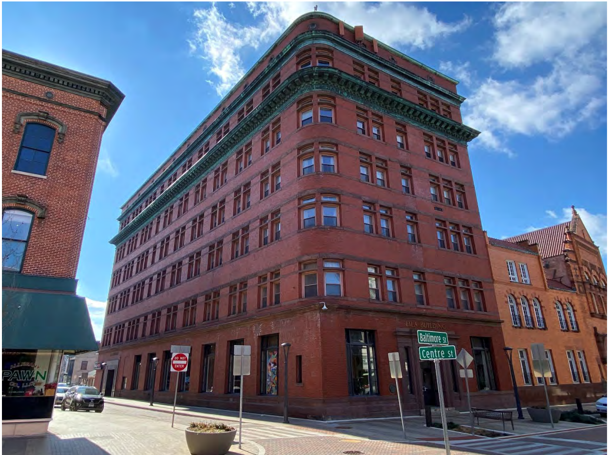
MD-Allegany_Cumberland Downtown Historic District Boundary Expansion_054 Photo 54 of 75. View of 83 Baltimore Street, looking southwest.
