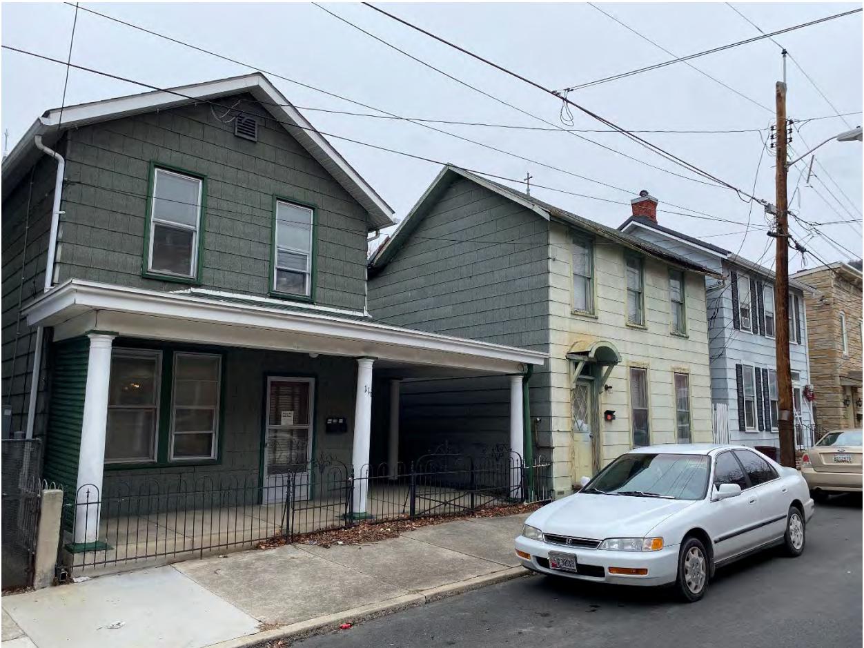
MD-Allegany_Cumberland Downtown Historic District Boundary Expansion_024 Photo 24 of 75. View of 118 & 116 Hanover Street, looking northwest.
