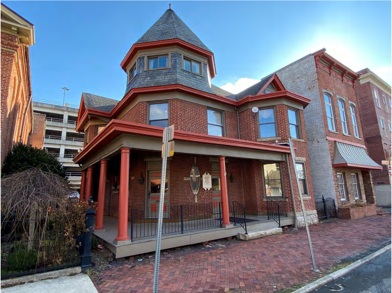
MD-Allegany_Cumberland Downtown Historic District Boundary Expansion_060 Photo 60 of 75. View of 110 South Centre Street, looking southeast.
