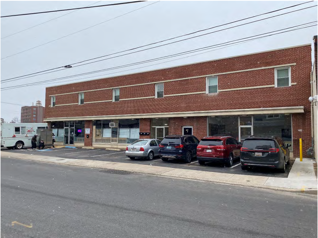
MD-Allegany_Cumberland Downtown Historic District Boundary Expansion_055 Photo 55 of 75. View of 130-134 North Mechanic Street, looking southwest.
