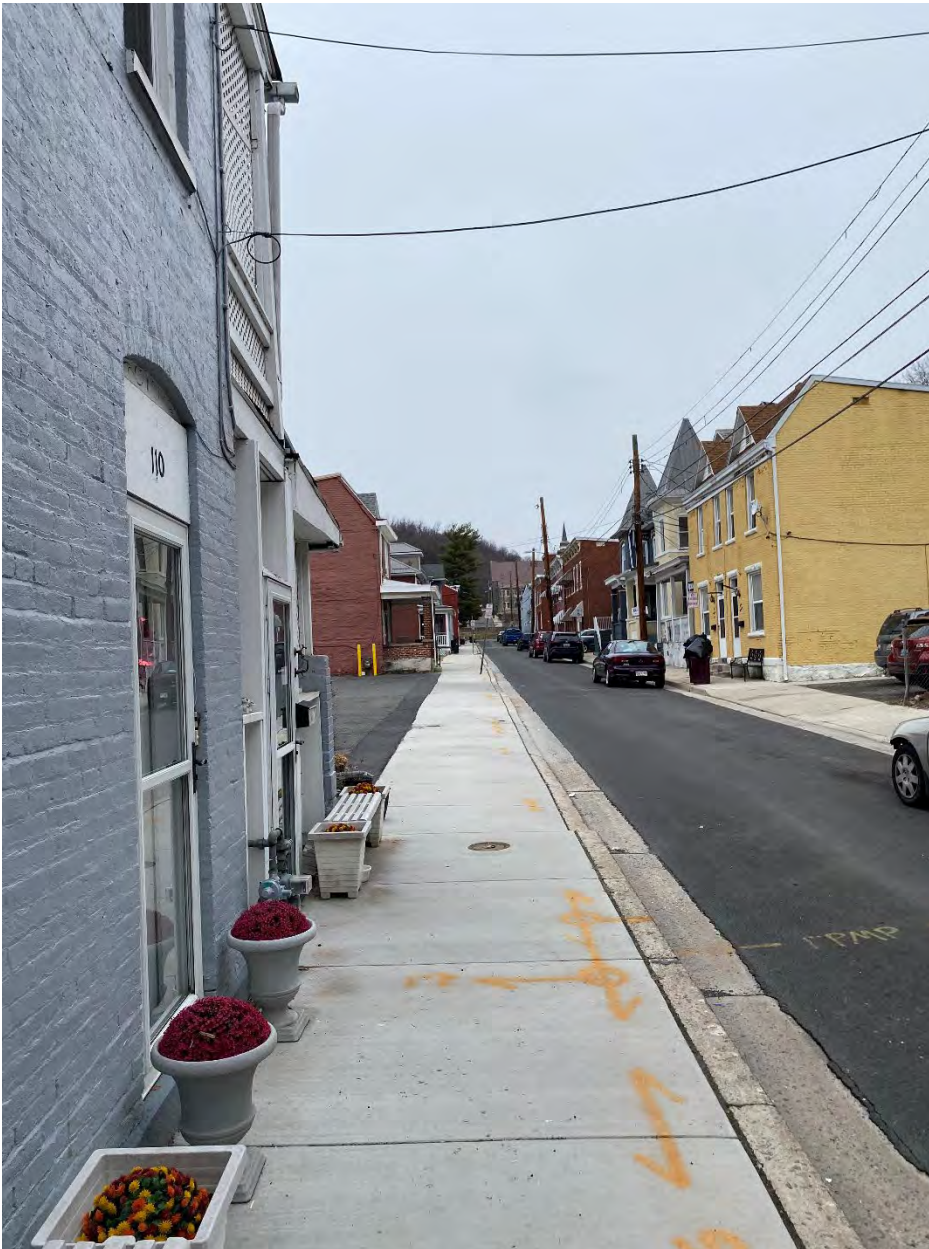
MD-Allegany_Cumberland Downtown Historic District Boundary Expansion_041 Photo 41 of 75. View to the north-northeast along Polk Street.
