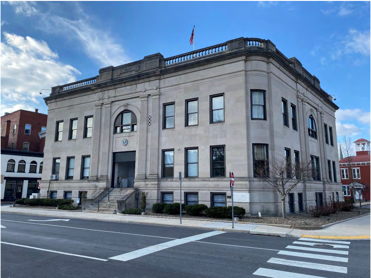
MD-Allegany_Cumberland Downtown Historic District Boundary Expansion_017 Photo 17 of 75. View of 57 North Liberty Street, looking southwest.
