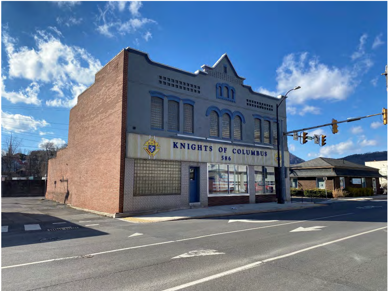
MD-Allegany_Cumberland Downtown Historic District Boundary Expansion_023 Photo 23 of 75. View of 66 North Mechanic Street, looking west-northwest.
