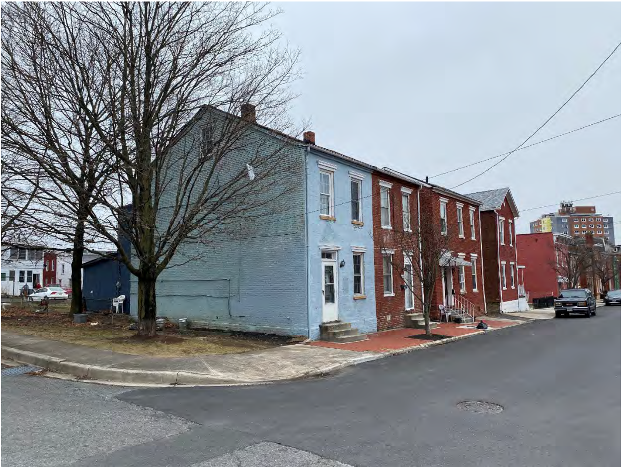
MD-Allegany_Cumberland Downtown Historic District Boundary Expansion_025 Photo 25 of 75. View to the west-southwest along Hanover Street.
