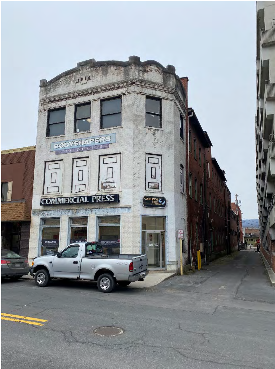
MD-Allegany_Cumberland Downtown Historic District Boundary Expansion_066 Photo 66 of 75. View of 109 South George Street, looking southwest.
