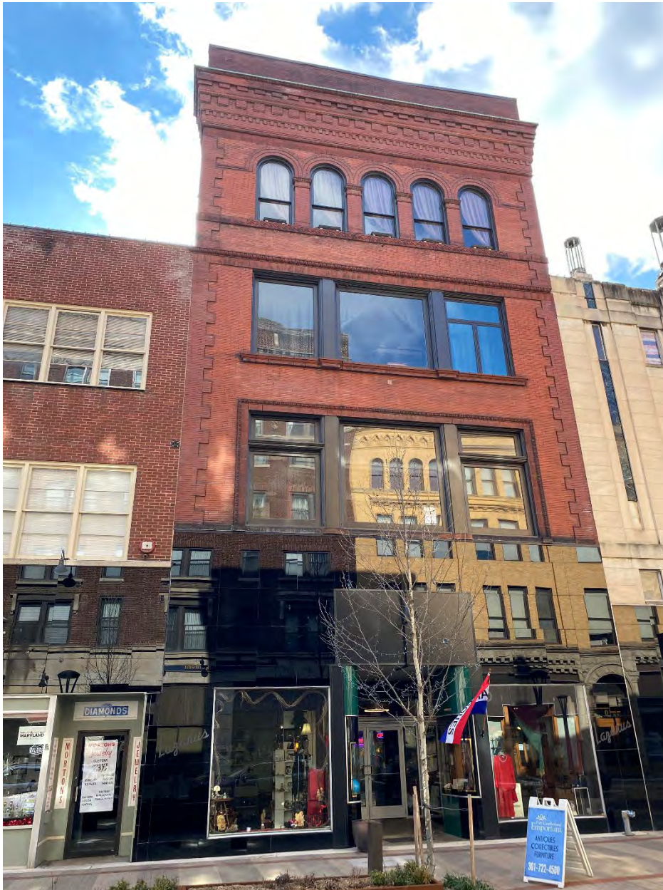
MD-Allegany_Cumberland Downtown Historic District Boundary Expansion_042 Photo 42 of 75. View of 55 Baltimore Street, looking south-southeast.
