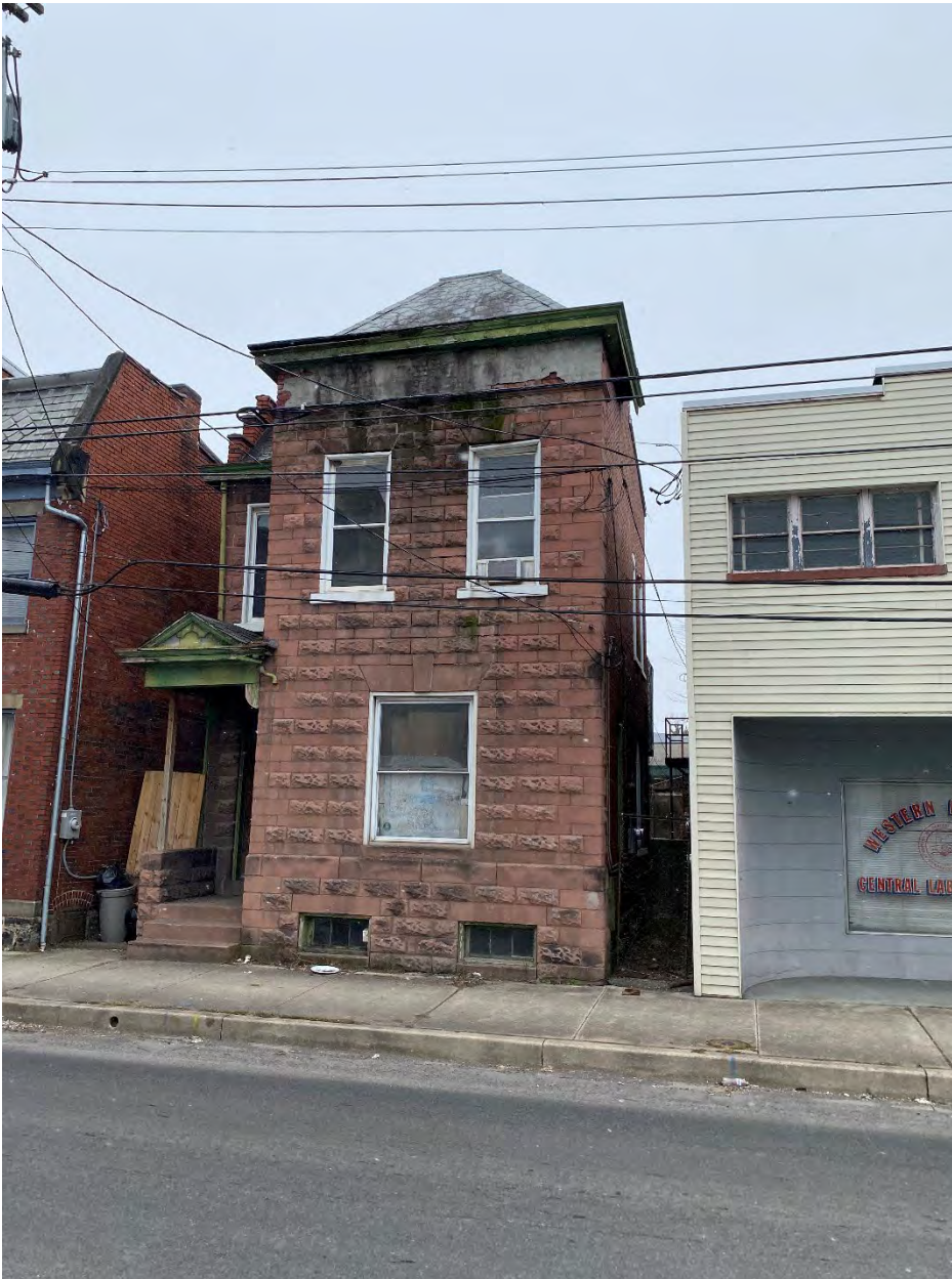
MD-Allegany_Cumberland Downtown Historic District Boundary Expansion_016 Photo 16 of 75. View of 150 North Mechanic Street, looking southwest.
