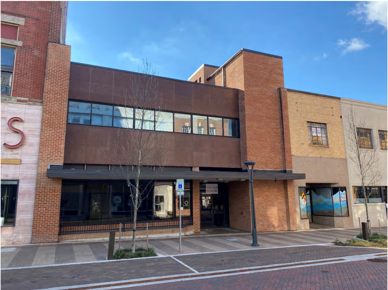
MD-Allegany_Cumberland Downtown Historic District Boundary Expansion_061 Photo 61 of 75. View of 141 Baltimore Street, looking southwest.
