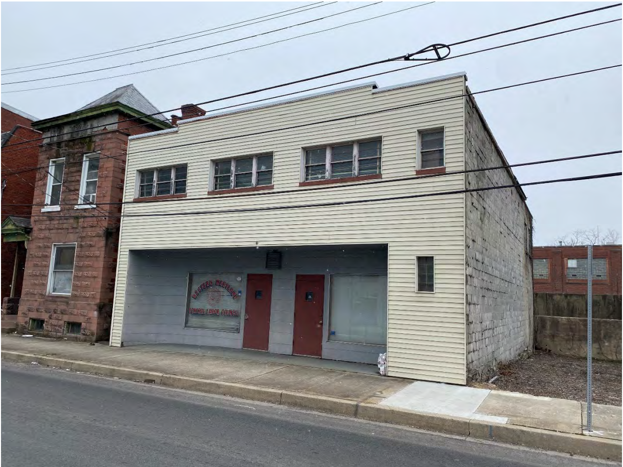
MD-Allegany_Cumberland Downtown Historic District Boundary Expansion_046 Photo 46 of 75. View of 152 North Mechanic Street, looking southwest.
