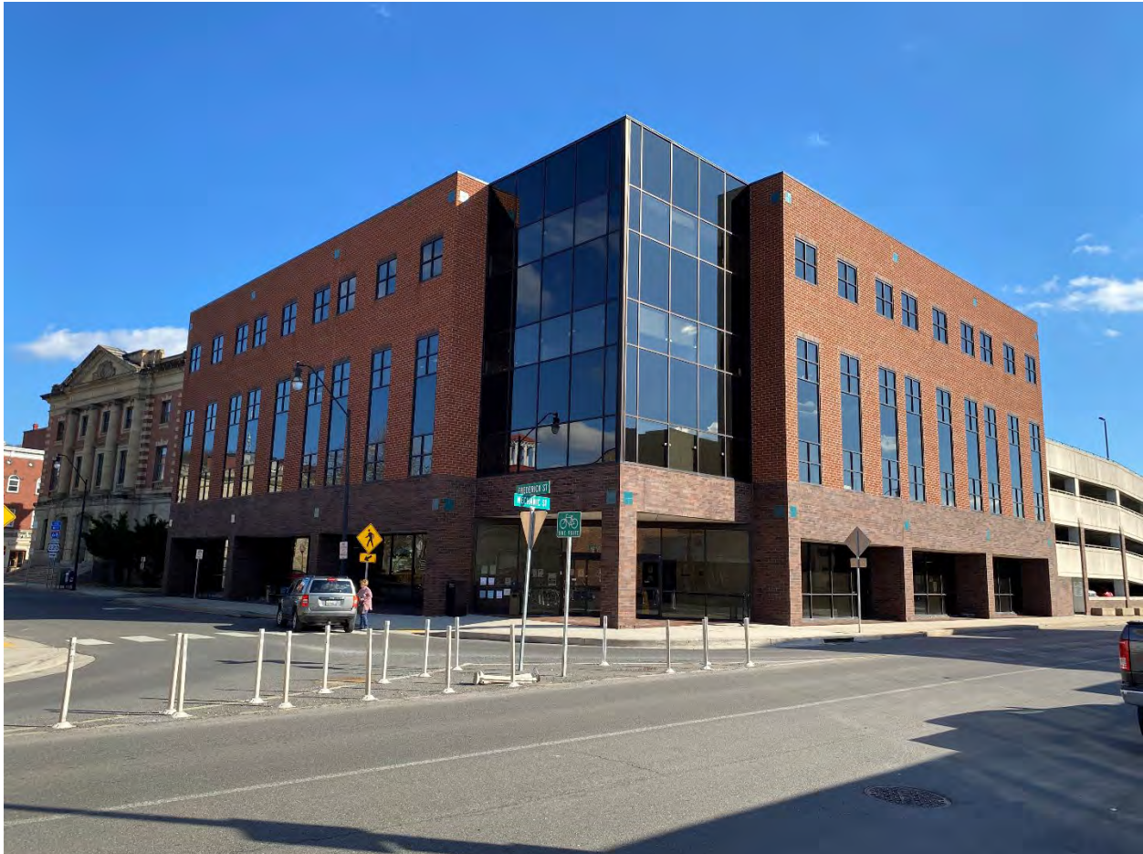
MD-Allegany_Cumberland Downtown Historic District Boundary Expansion_020 Photo 20 of 75. View of 1 Frederick Street, looking southeast.
