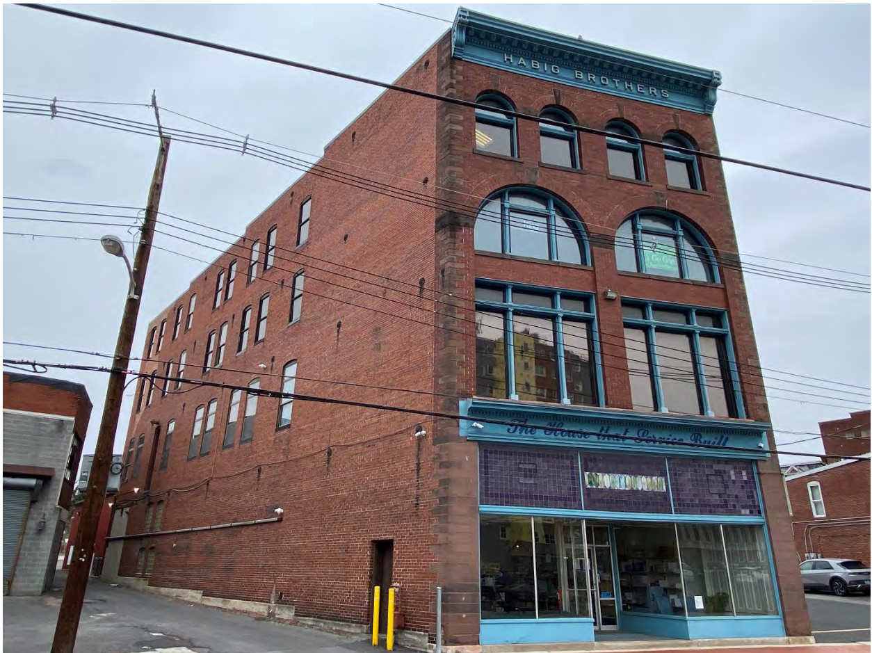
MD-Allegany_Cumberland Downtown Historic District Boundary Expansion_071 Photo 71 of 75. View of 151 North Centre Street, looking east-southeast.
