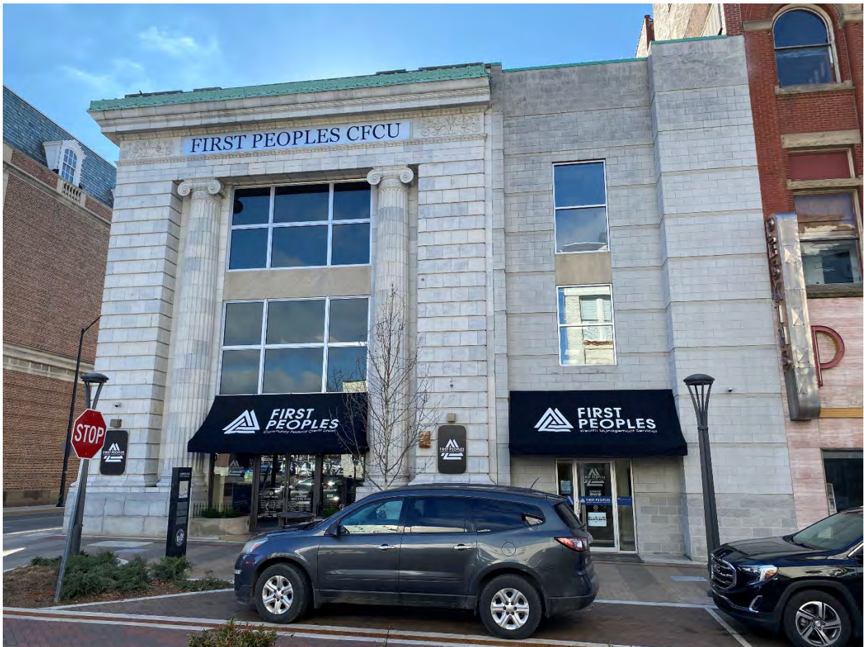
MD-Allegany_Cumberland Downtown Historic District Boundary Expansion_010 Photo 10 of 75. View of 149-153 Baltimore Street, looking south-southeast.
