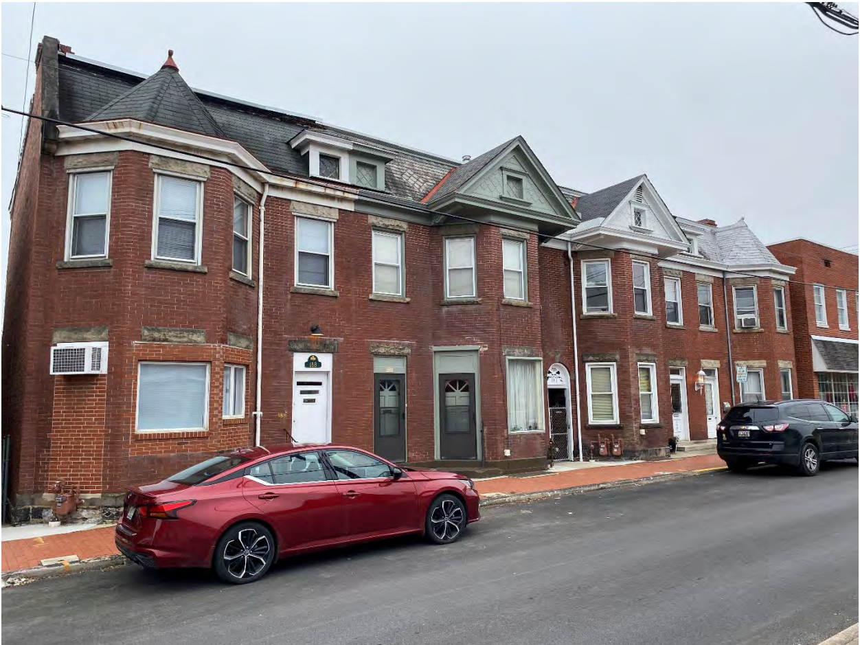
MD-Allegany_Cumberland Downtown Historic District Boundary Expansion_015 Photo 15 of 75. View of 188-194 North Centre Street, looking west.
