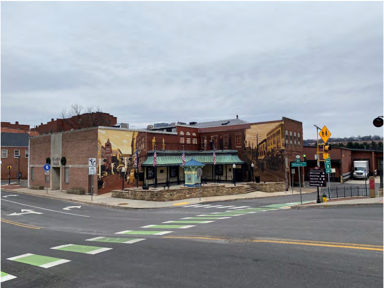
MD-Allegany_Cumberland Downtown Historic District Boundary Expansion_019 Photo 19 of 75. View of 19 Baltimore Street, looking southwest.
