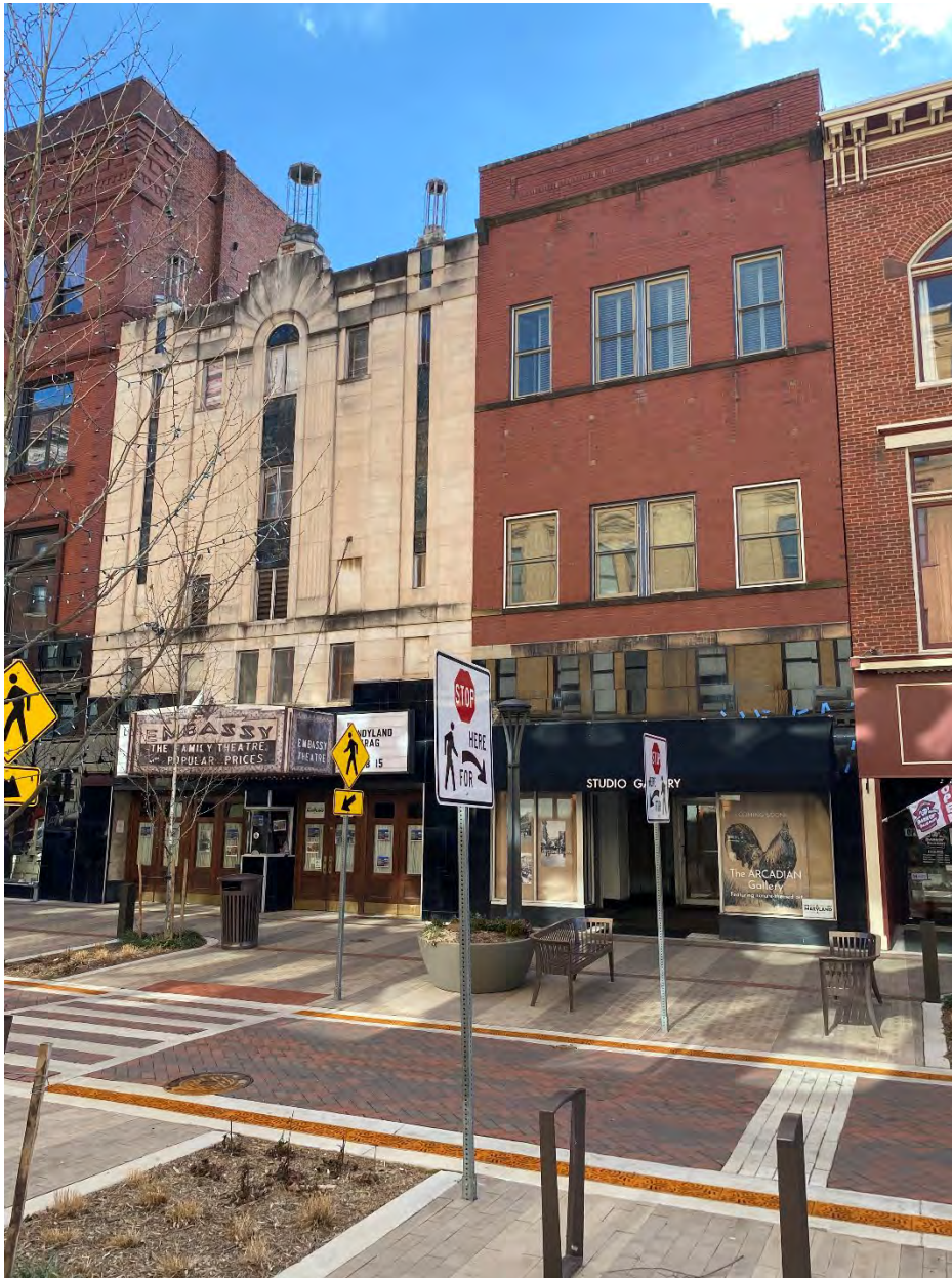
MD-Allegany_Cumberland Downtown Historic District Boundary Expansion_013 Photo 13 of 75. View of 47 & 49 Baltimore Street, looking southeast.
