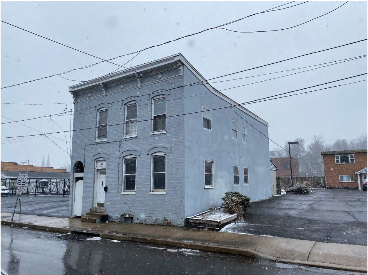
MD-Allegany_Cumberland Downtown Historic District Boundary Expansion_034 Photo 34 of 75. View of 240 North Mechanic Street, looking southwest.
