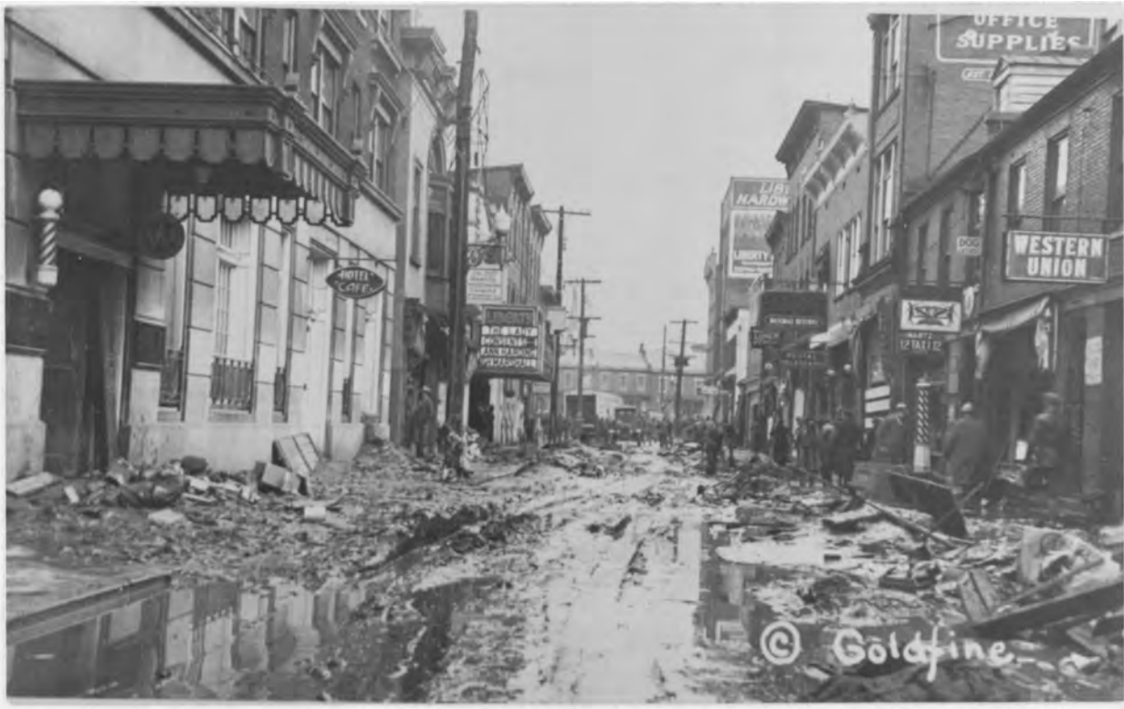
Figure 7. The aftermath of the St. Patrick's Day Flood of 1936, looking north along North Liberty Street.
