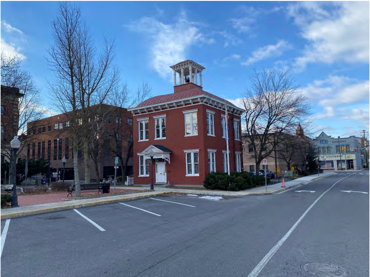
MD-Allegany_Cumberland Downtown Historic District Boundary Expansion_002 Photo 2 of 75. View of 24 Frederick Street, looking southwest.
