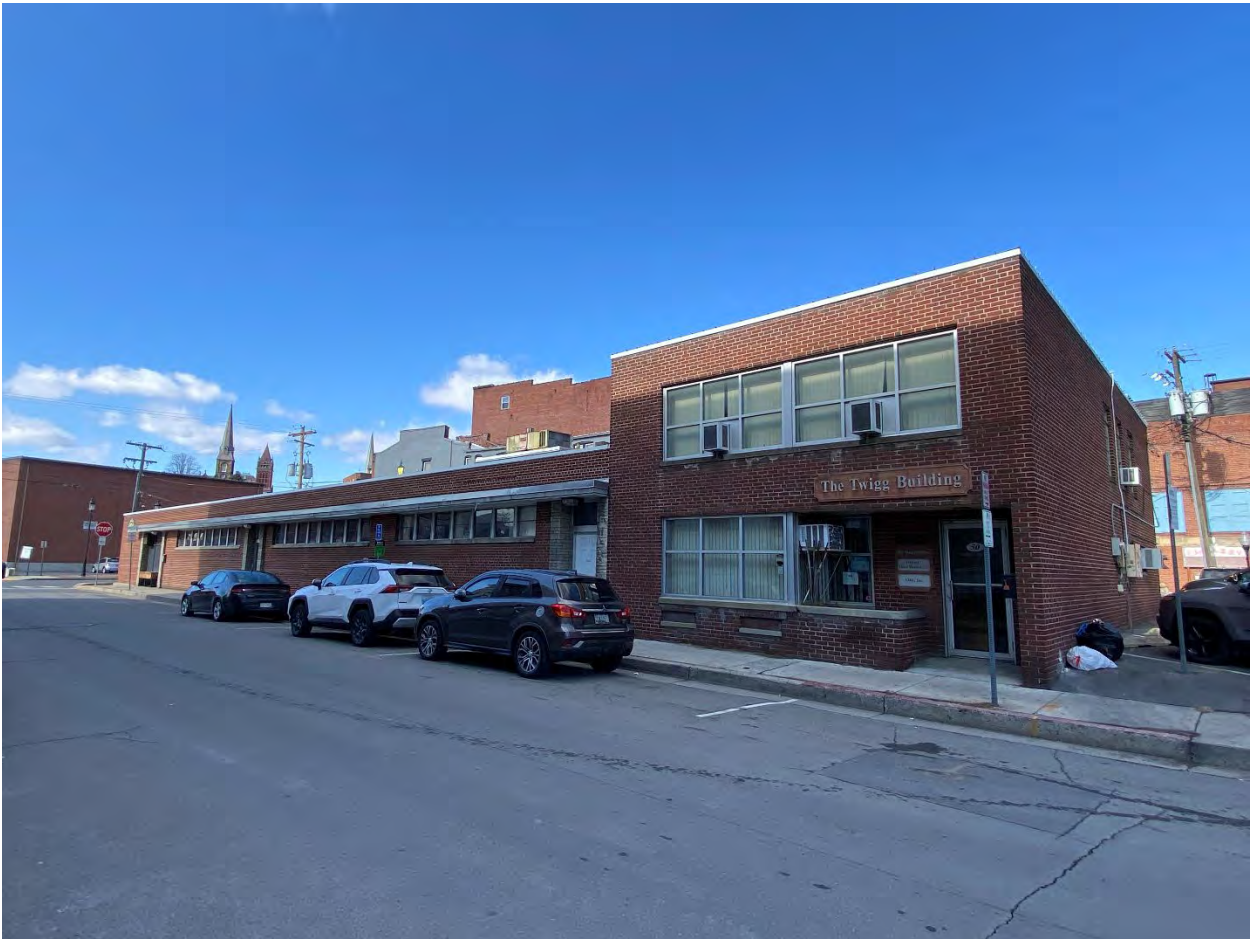
MD-Allegany_Cumberland Downtown Historic District Boundary Expansion_045 Photo 45 of 75. View of 20-50 Pershing Street, looking west-northwest.
