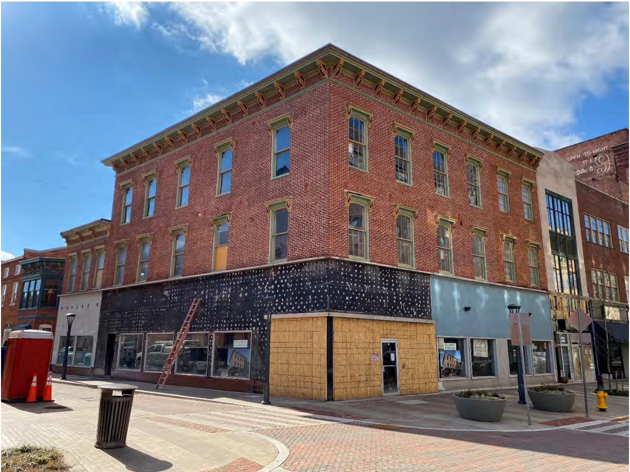
MD-Allegany_Cumberland Downtown Historic District Boundary Expansion_004 Photo 4 of 75. View of 69 Baltimore Street, looking southwest.
