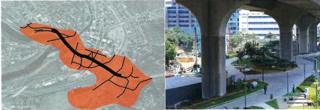
An enormous share of the downtown's land is affected by the I-68 viaduct and its ramps. Structural redesign of the highway including can reduce footprint of the structure that keeps a large swath of land in the shadows.
