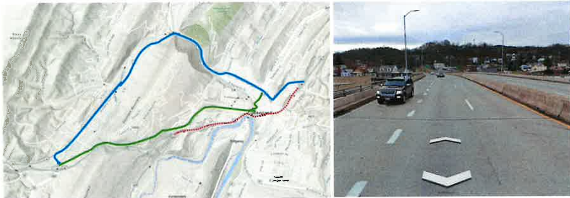
I-68, the "National Freeway," runs on an elevated structure through Cumberland. It is in significant need of structural repair which brings both challenges and opportunities for the city.
