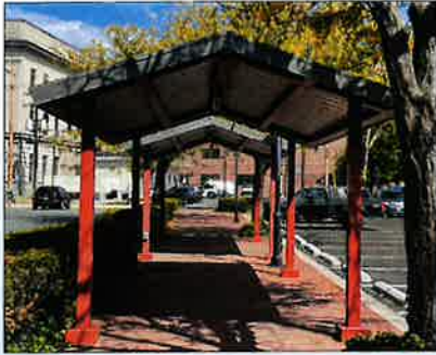
Downtown Pedestrian Connection Existing Structure Reference
